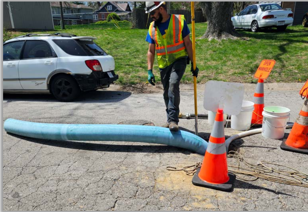
Sewer Relining Process
